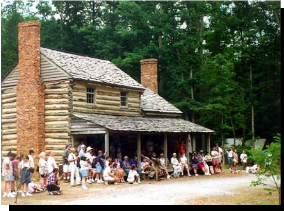
The Hofauger House, a historical farmhouse (circa 1837), was reconstructed in 1991 at Virginia's Explore Park.
